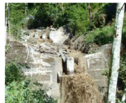
crash dams - compound barrier (Klemmgraben, Salzburg, Austria)
