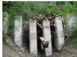
debris flow breaker - Sectional barriers with fins (Kreuzgraben, Salzburg)
